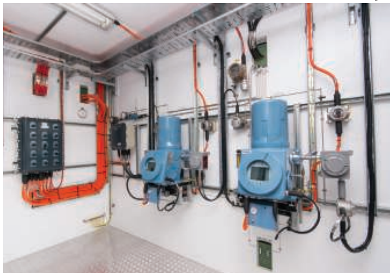
FIGURE 4. Gas chromatograph software control of a gas chromatograph is easier with intuitive, Windows-based pulldown menus and fill-in-the-blank tables. The software collects and organizes the analyzed data from gas chromatographs, such as the 700XA model shown here
